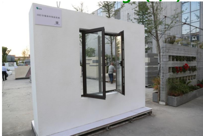
Printed Wall Integrated with Door and Window
