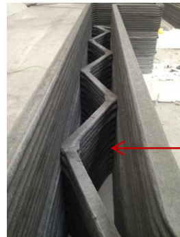
Hollow Wall Save Cost Place Pipes Thermal Insulation
