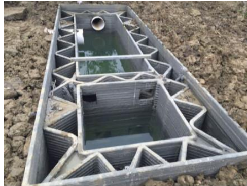
Installation of 3D Printed Tank
