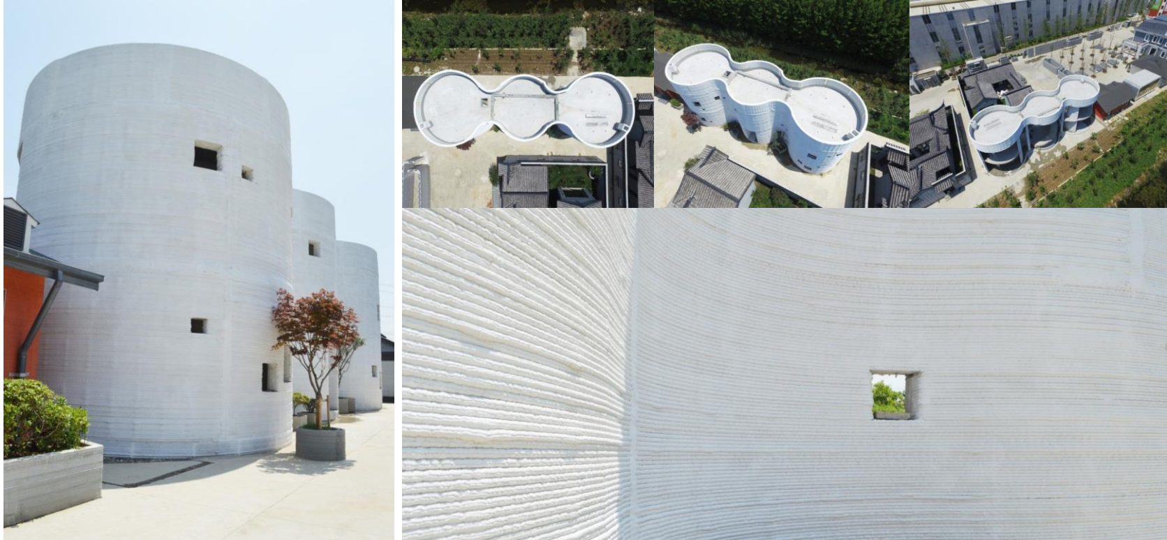
3D-printed undulated building
